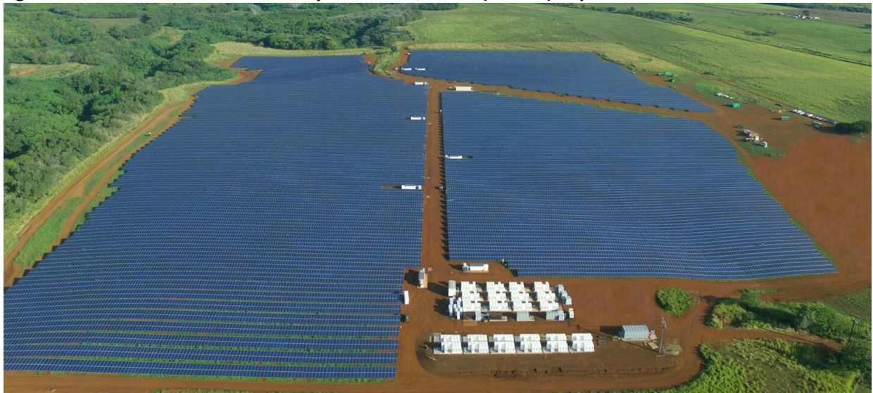
Figure 3-17: Photo of the PV + battery solar farm/TESLA (Hawaii) Kapaia Installation
